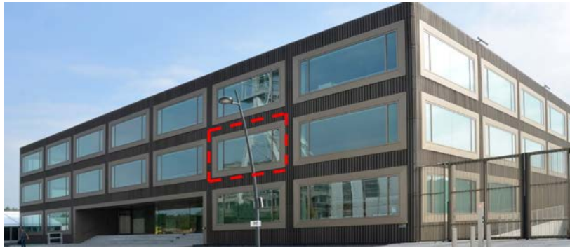
Figure 3-8 EnergyVille 1, Thor Park 8310, 3600 Genk
